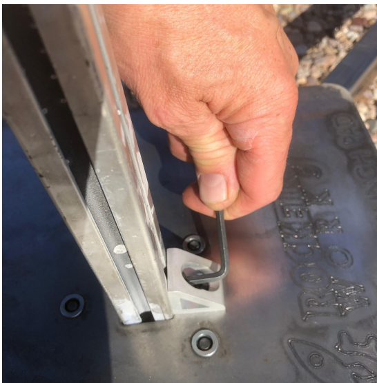
Tightening the rail against the angle bracket provides the tension that produces stability.
